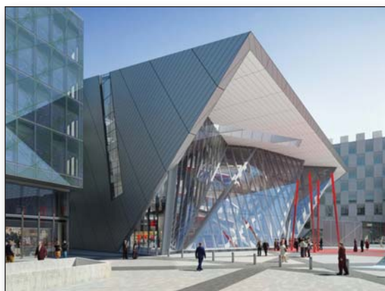
Yet another startling new addition to the Dublin product is the Grand Canal Theatre. Seating 2,100 this iconic building was designed by world renowned architect Daniel Libeskind. It will be Ireland's leading touring theatre for musicals, ballet, family shows, drama, concerts, and opera. It has the largest theatre stage in Ireland, and opens the door to large theatrical productions which were previously unable to visit here.
