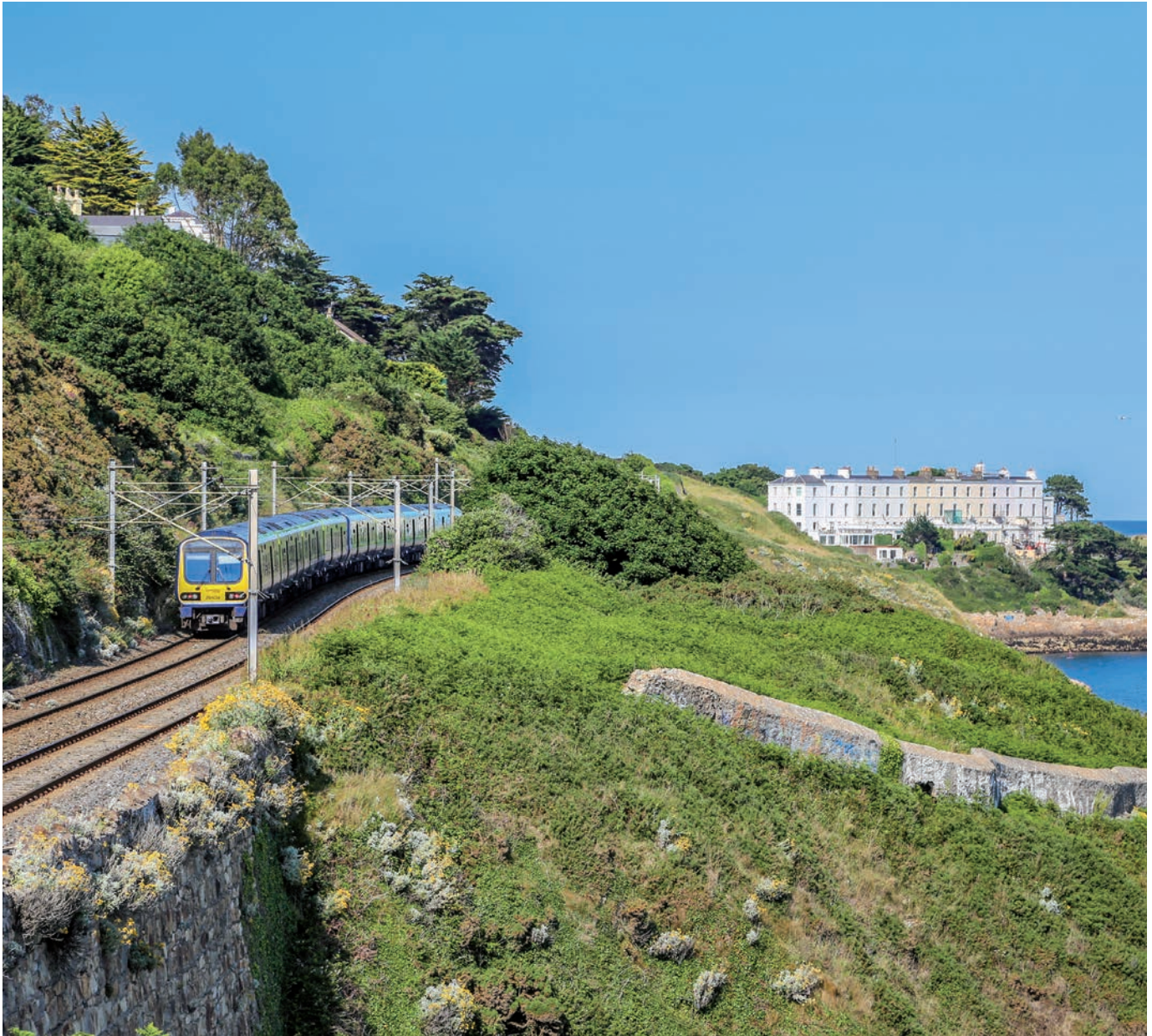
Railway Line - Killiney, Co. Dublin
